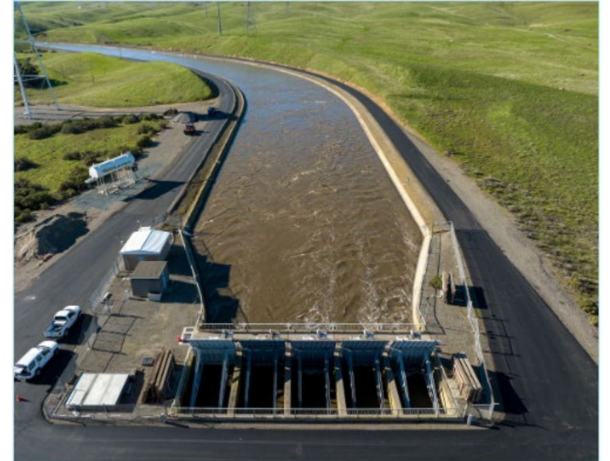
A drone provides a view of water pumped from the Harvey O. Banks Delta Pumping Plant into the California Aqueduct at 9,790 cubic feet per second after January storms. Photo taken January 20, 2023.
